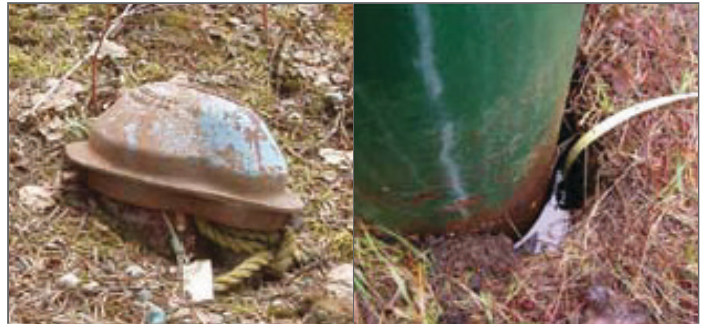
FIGURE 1 Well casing stickup less than 30 cm (1ft) from the ground surface
