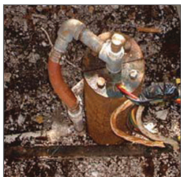
FIGURE 5 Well with sanitary seal type cap
